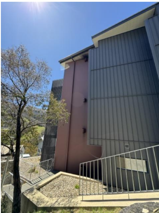
Figure 5 & 6: Side elevations. Note red cladding to be replaced.
