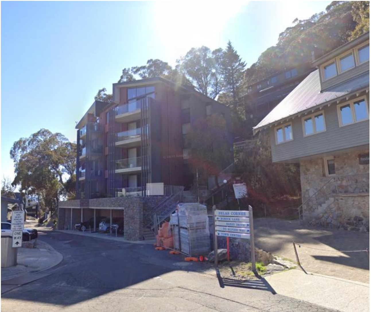
Figure 2: The subject site. Note red cladding to be replaced.
